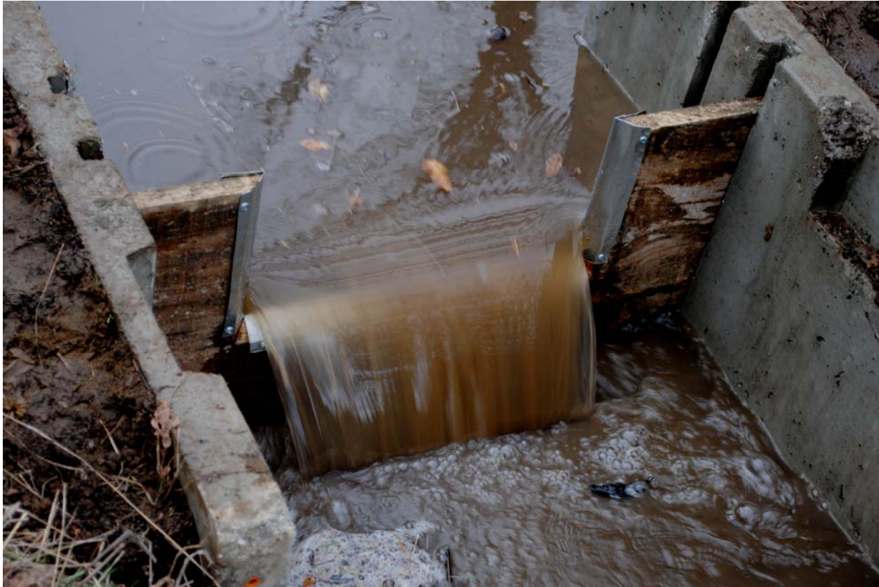
Figure 7. Installed Rectangular Weir.
