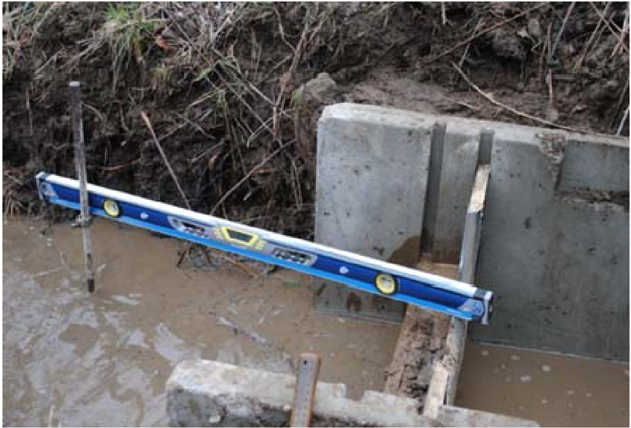
Figure 5. Leveling the witness post to the weir crest.
