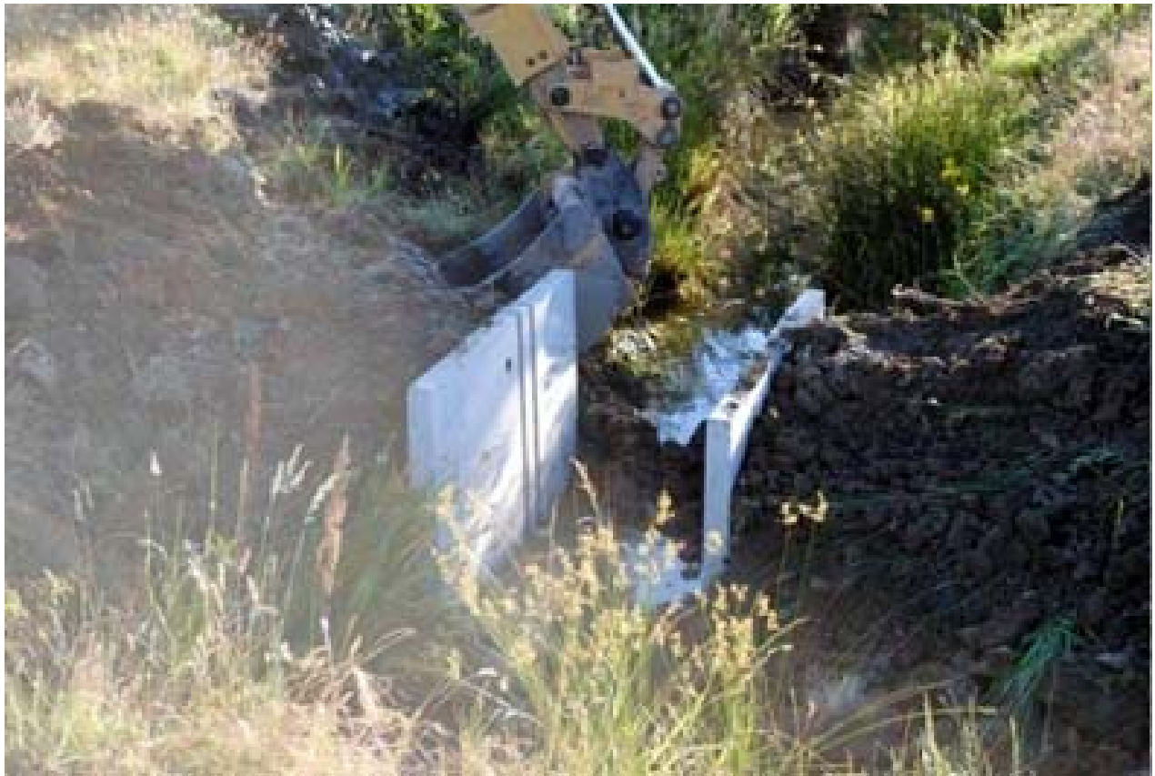
Figure 2. Setting a precast weir box with a backhoe.
