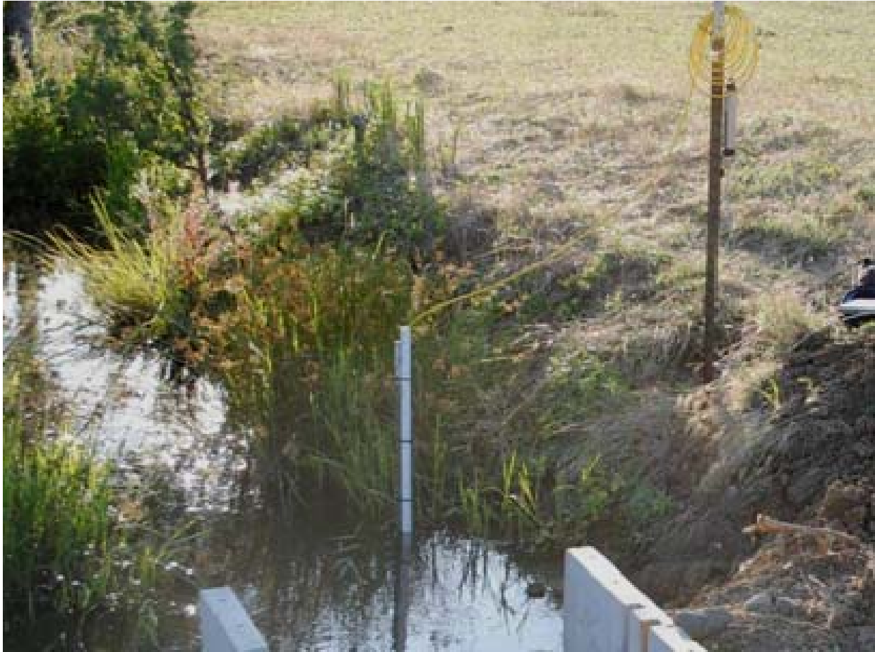
Figure 6. Demonstrates typical installation of pressure transducer.
