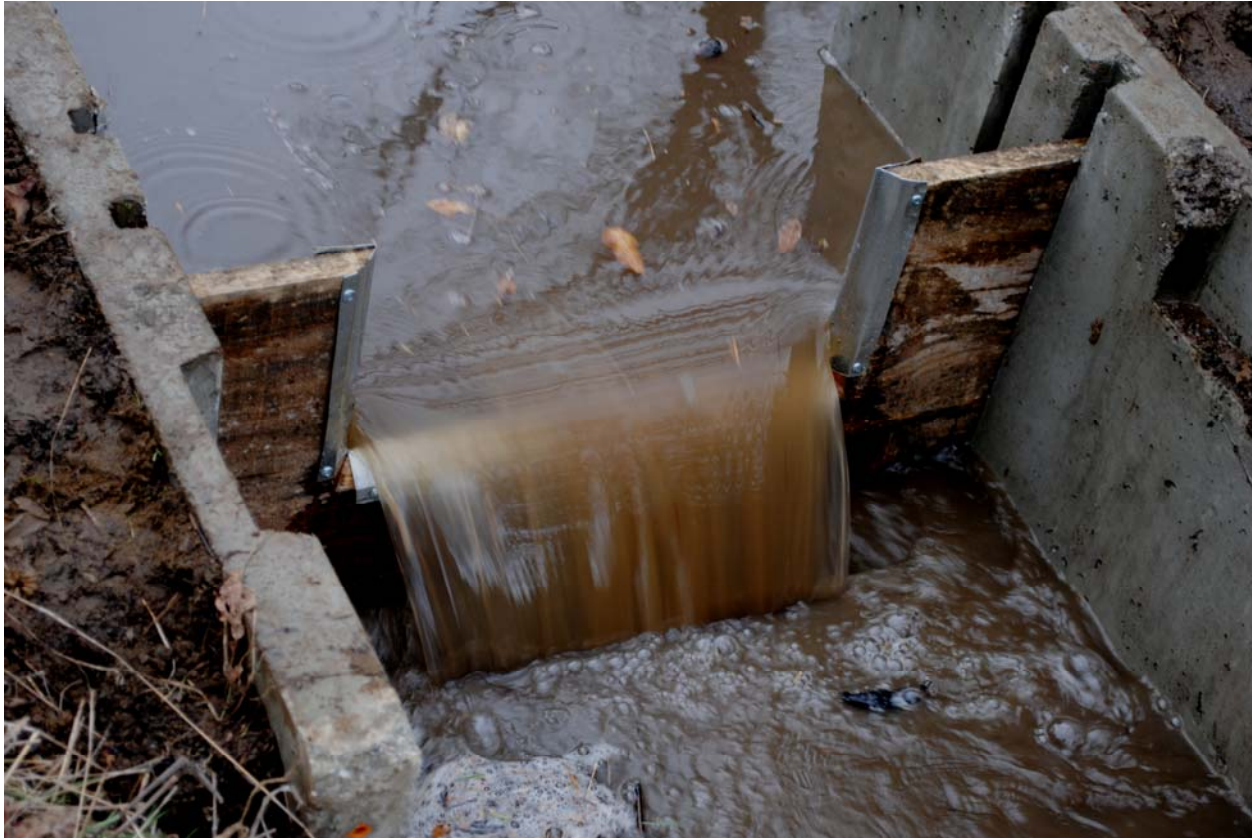
Figure 7. Installed Rectangular Weir.
